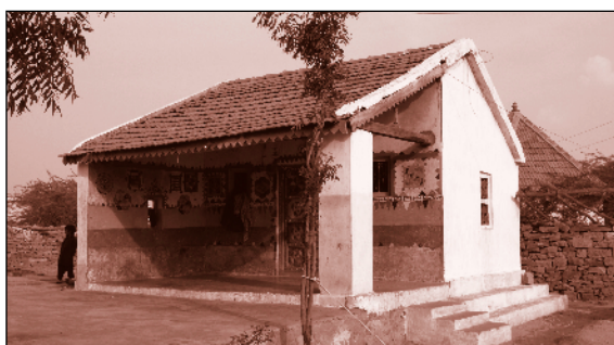
Owner-built houses in Gujarat
